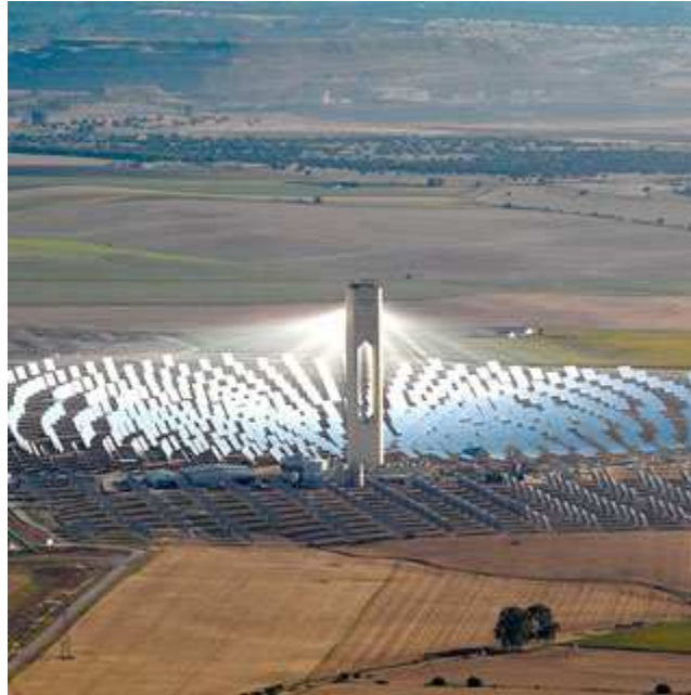
Figure 5-21 Solar power tower plant
