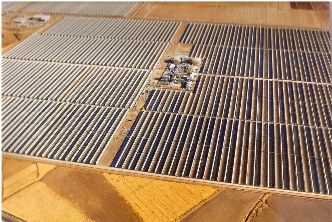
Figure 5-19 Parabolic trough solar
