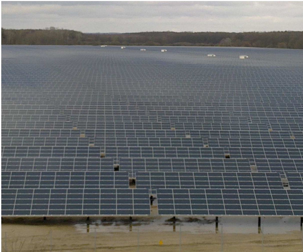
Figure 5-5 Utility great scale photovoltaic power plant
