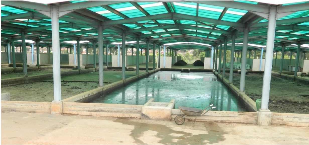
Figure 3-12; Faecal sludge drying beds at Lubigi treatment plant, Uganda Source: Author
