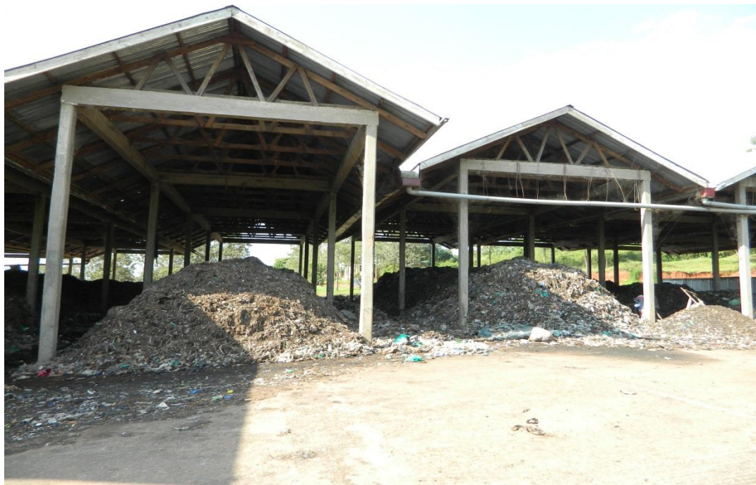
Figure 3-13: Composting section within Mukono Town Landfill.
